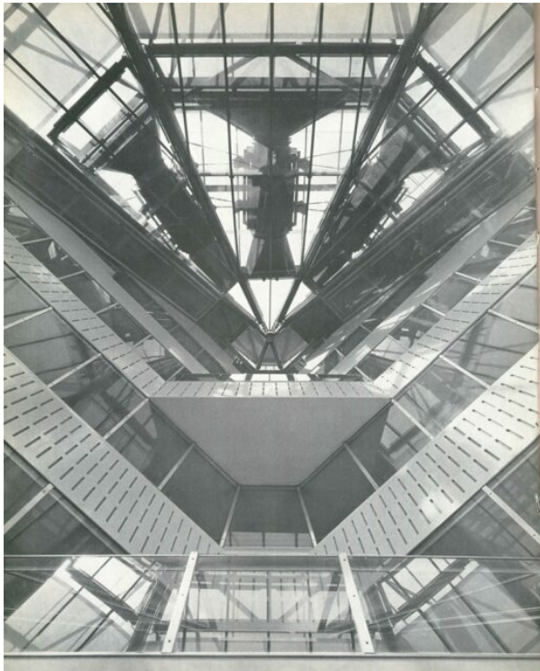
Opposite: the vertical axis runs the apex of the reading room of the History Faculty bridge together the essential elements of the design, the ventilating fins of the roof are an environmental feature, and the access galleries to the two teaching rooms that form the two arms of the glass enclosing the library.
